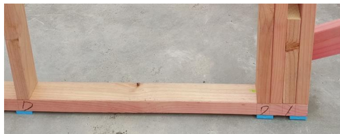
Double door studs only require one packer, Stud block stud only require one Packer.
